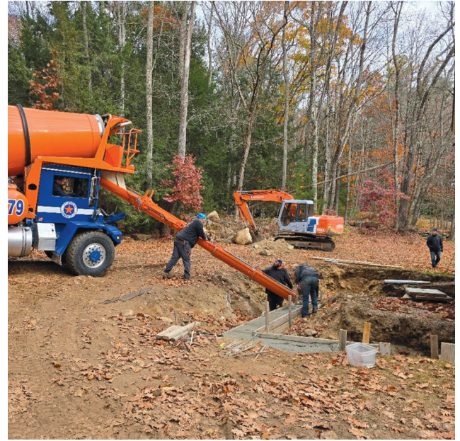
Pouring the footings (by 413 Concrete) with CW Nelson's Excavator in the background.
